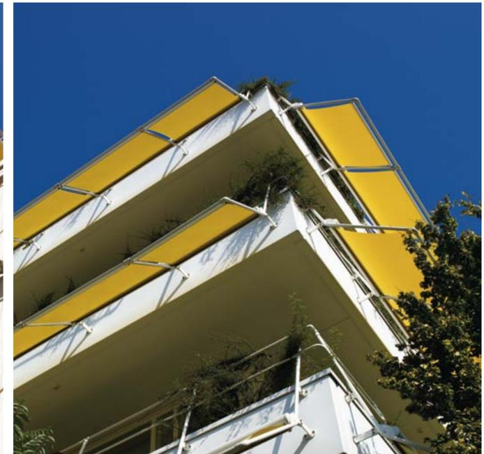
The sun shade system is both beautiful and intelligent. Its sophisticated design contributes to eliminating glare effects in the spaces without blocking the view when in use. The view outside remains unobstructed. This significantly increases the potential of the rooms, which is also reflected in the well-being of the employees.
